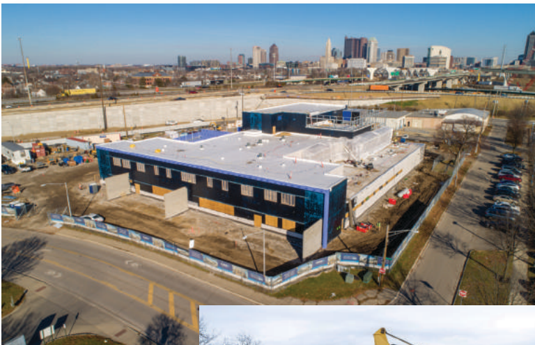
Drone photo shows construction progress as of December 2023.
